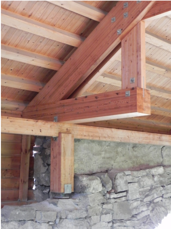
Figure 3: Laminated lumber post bearing on existing rubble wall.
