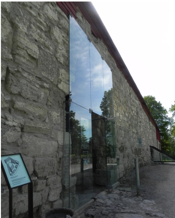
Figure 2: Detail, west facade, primary entrance.
