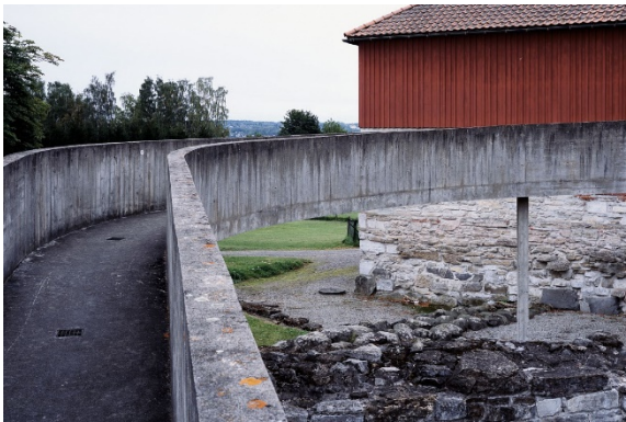
Figure 4: Cast concrete ramp curving above excavations at court.
