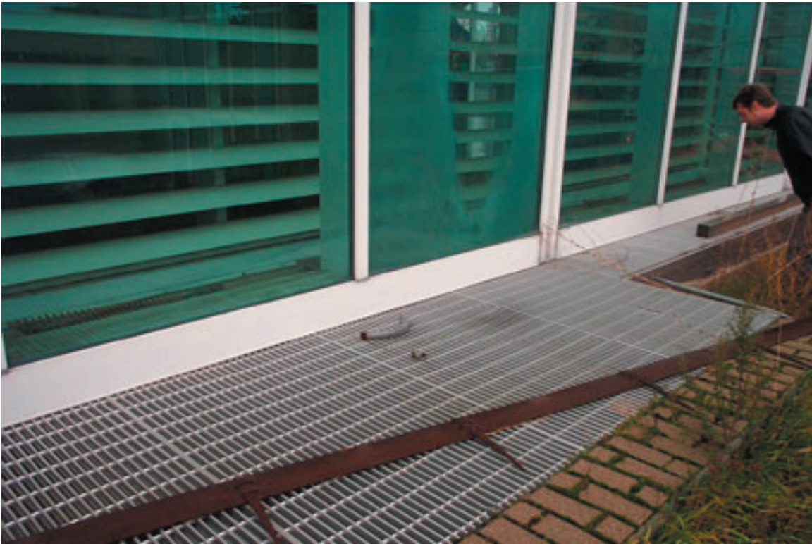
View of air intake grille at base of building. Note clouding on center glazed unit.
