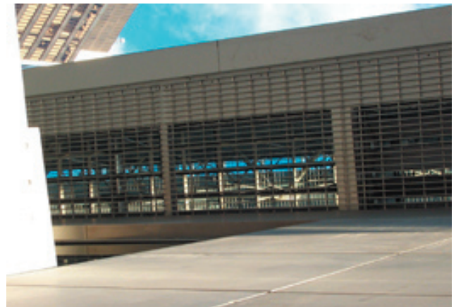
Summer Wall Section: Dampers Open
