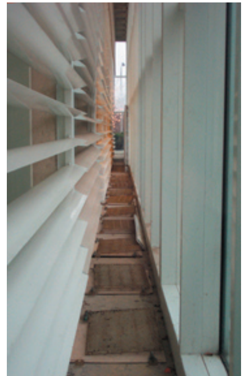
A view inside the cavity showing its clear width to allow for maintenance; the plywood sheets that close off the grille at the base preventing air intake.
