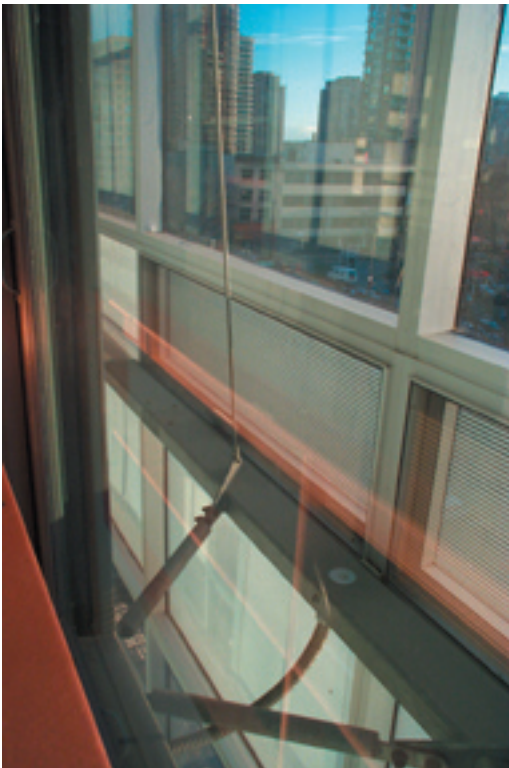
Views looking into the cavity. Note the differentiated glazing materials: clear and fritted, as well as the operable window.
